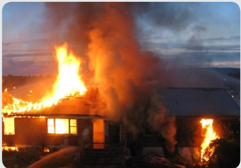
The roof on the right was coated with HybridSil™
