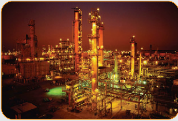
Curtiss-Wright supplies critical components to chemical processing plants around the world.
