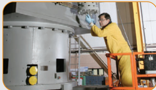
Factory service is performed by a CW employee on one of the 300+ motors supplied to over 100 nuclear power plants worldwide.
